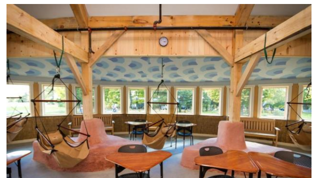
Figure 3: Colby-Sawyer College's Sunshack (inside view of cob benches and concrete floors which add thermal mass).
