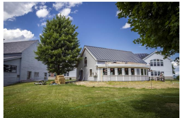
Figure 4: Colby-Sawyer College's Sunshack (outside view). This building was built by students, faculty, and volunteers. Today, it is a sustainable classroom.
