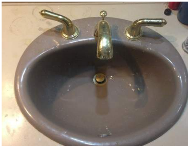
Ring dirt stains above the handles, toothpaste stains on the spout and handles
