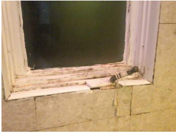
It is really hard to keep mold and dirt build up out of this area of the shower
